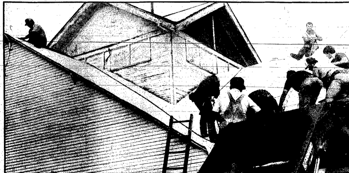
VOLUNTEERS HELP nail down fiberglass sheets, donated by Timpt, Inc., to the agriculture hall at the Wayne County Fairgrounds. For the past five weeks, workers have been meeting Tuesday night to complete the roof project. Approximately 30 volunteers assisted in the project.
